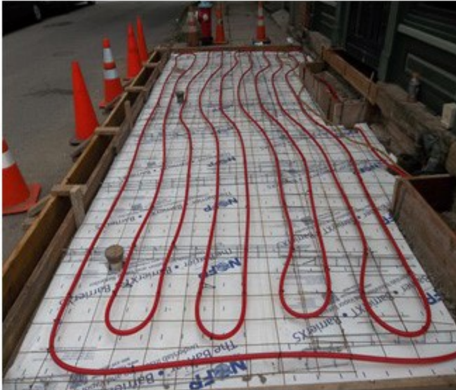
Snow Melt System installed by Phillips Heating.
