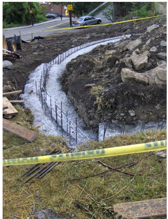
July 12, 2007 – substructure poured. (view from Monastery)
